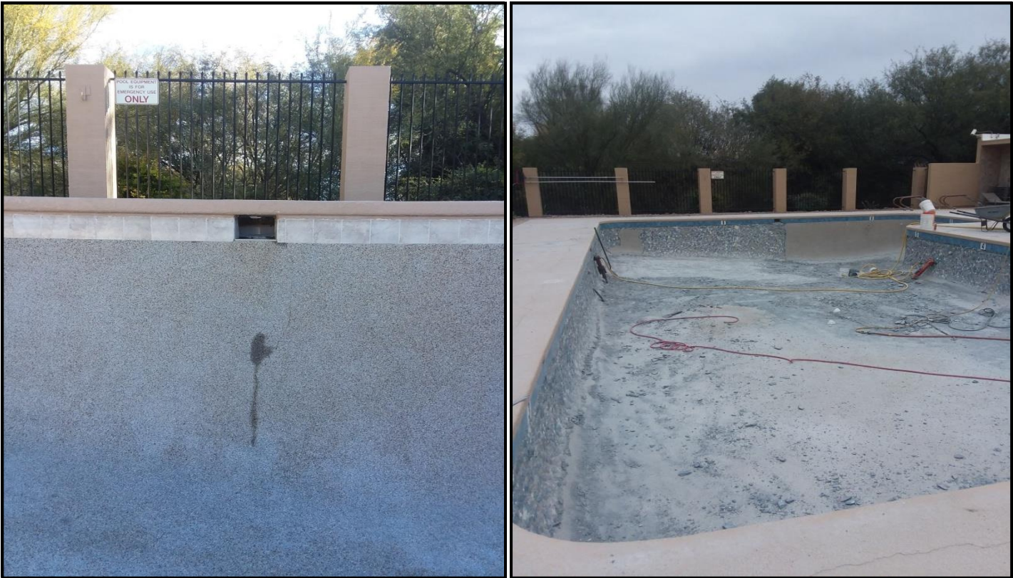
Crack on east wall of pool (not first crack of May 15) Removal of the Pebble Tech
