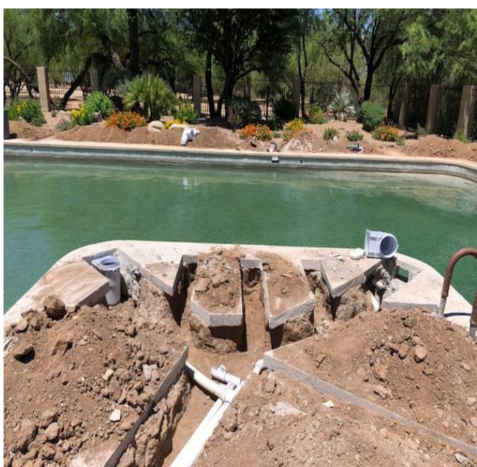
Laying out the pipes
