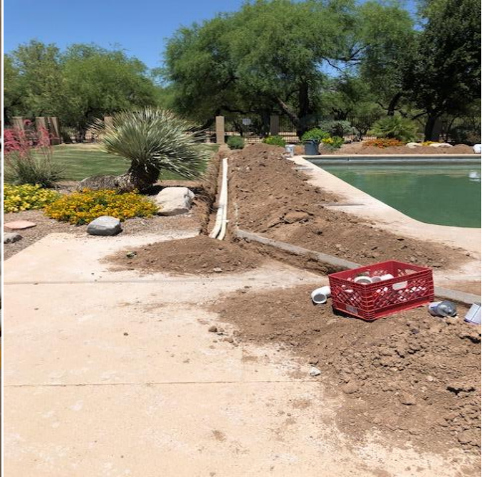
Laying out the pipes
