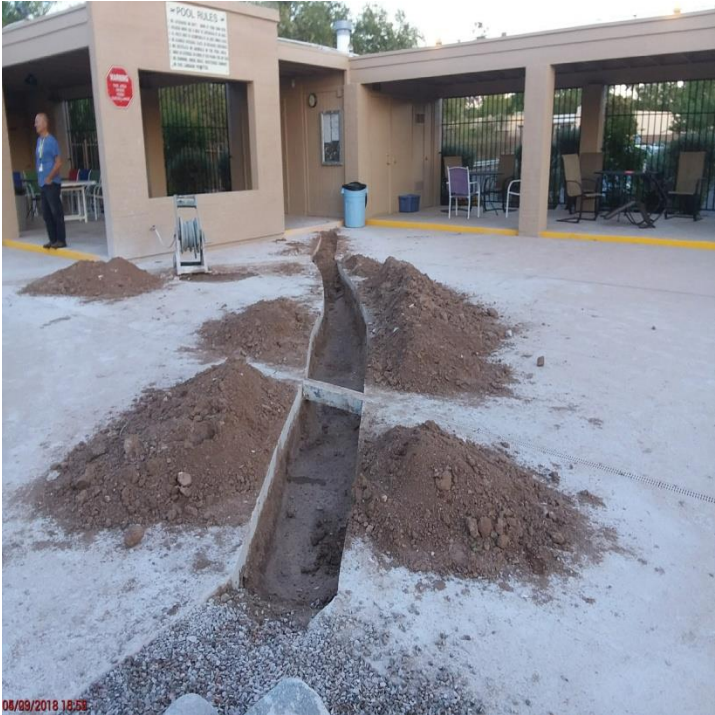
Trench to the equipment room,
