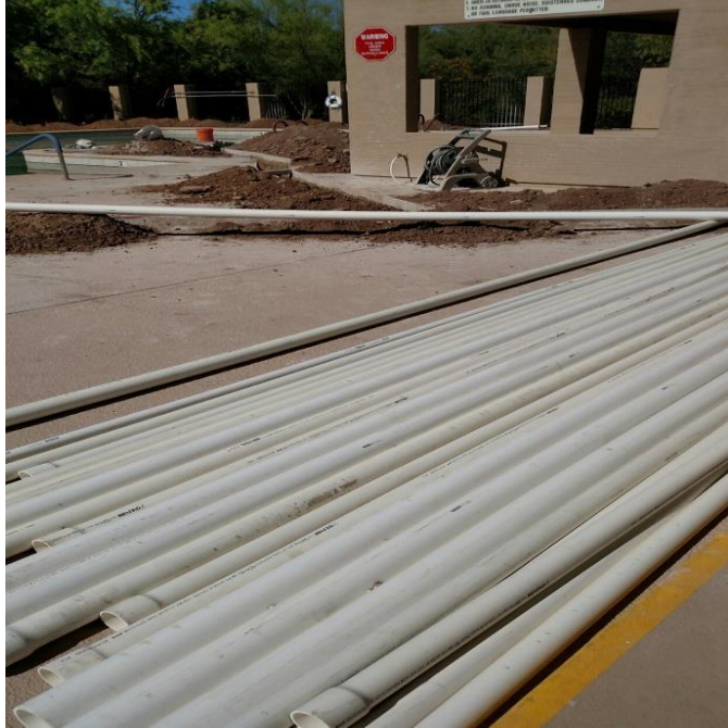
The new suction and pressure pipes.
